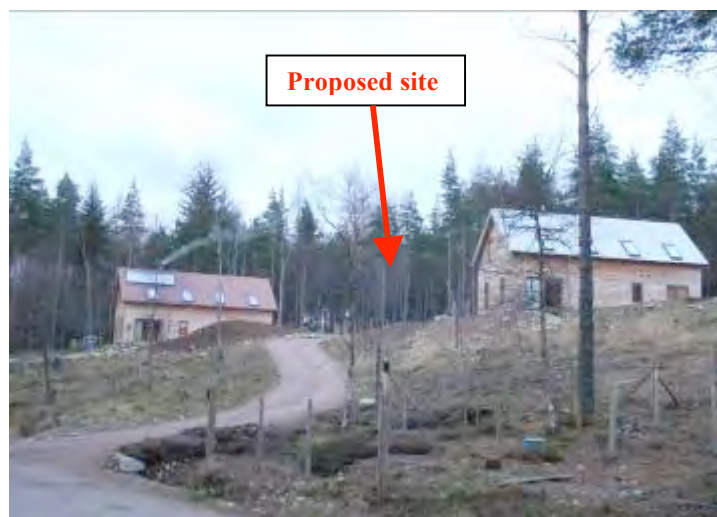
Fig. 2 : Existing access track serving Phase I dwellings
